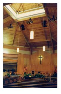
Glued laminated and heavy timber structures allow for large open spans and the beauty of exposed wood, a combination sure to enhance the experience of the structure.
